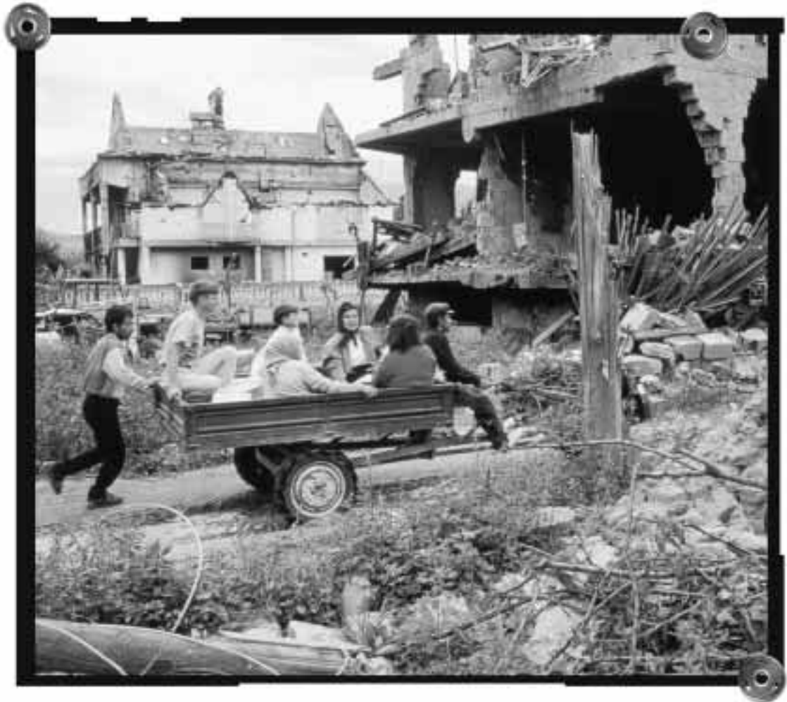
Returns arrive at their heavily damaged homes or schools in Mitrovica, Kosovo. UNHCR/06.1999/R. LeMoyné
